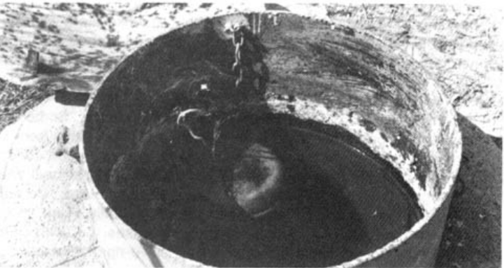
Float-valve regulates water level in stock tank.
